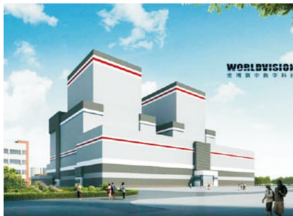
Shenhua Baoqing Power Plant
