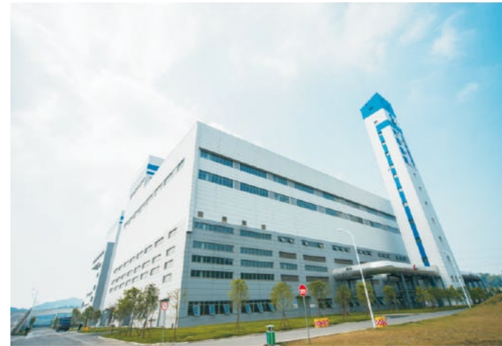
Chengdu Wanxing Environmental Protection Power Plant
