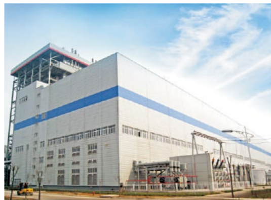
Anyang Power Plant
