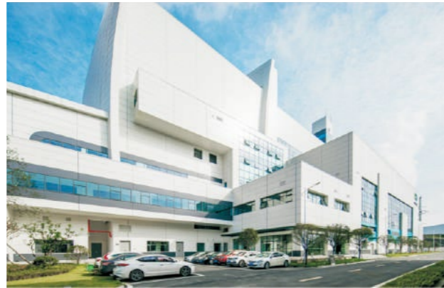
China Energy Saving Jintang Waste Power Plant
