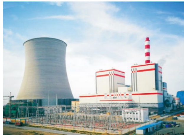
Xinjiang Korla Power Plant
