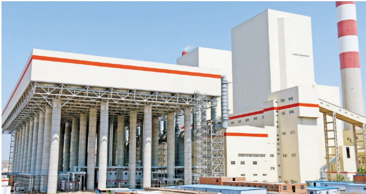
Shimizugawa Power Plant
