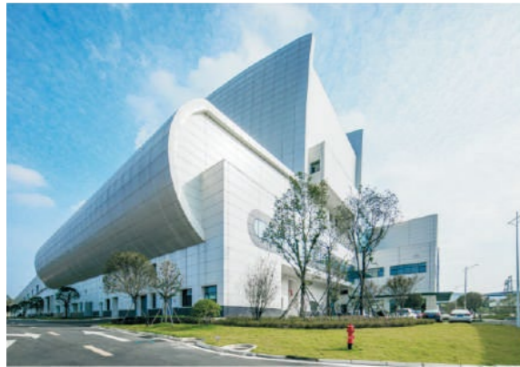
China Energy Saving Jintang Waste Power Plant
